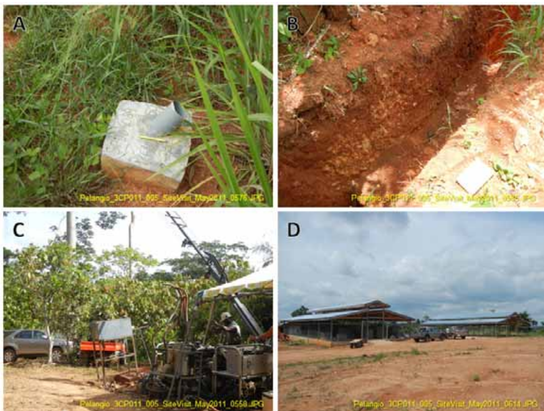
Figure 14: Exploration, Trenching and Drilling Activities on the Manfo Project.
